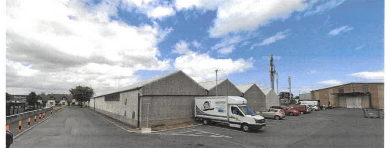
View looking at the existing South Eastern site boundary at the rear of the site
